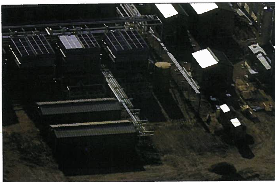
The injection pumps are in the two long buildings in the lower left. The pipe rack coming out of pump buildings goes towards the aerial compressor coolers. Two variable-frequency-drive buildings are to the right of the pump buildings. Two transformers are behind the VFD buildings. The Heatric exchangers' open skid is visible behind the pump-skid building (Fig. 1).
